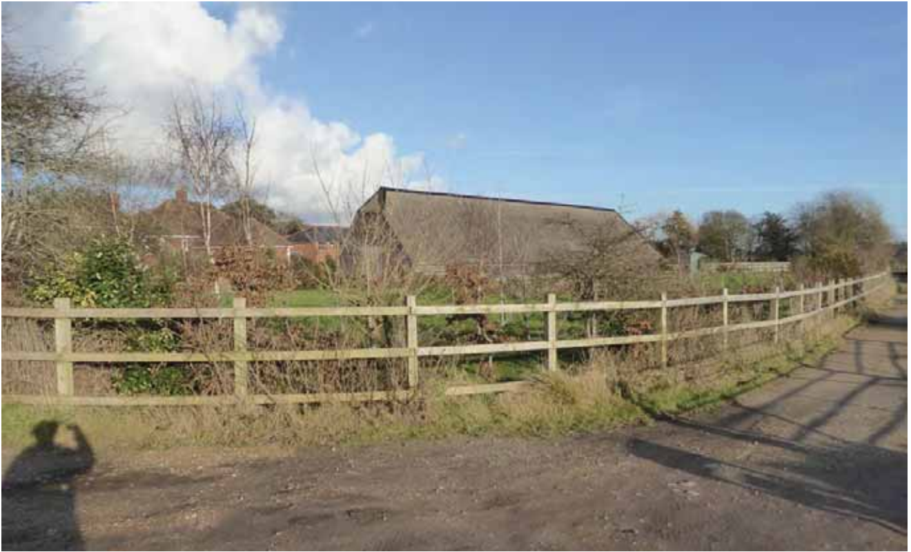
Appendix 7.1: The southern barn, from the south-west at the access road off Posbrook Lane.
