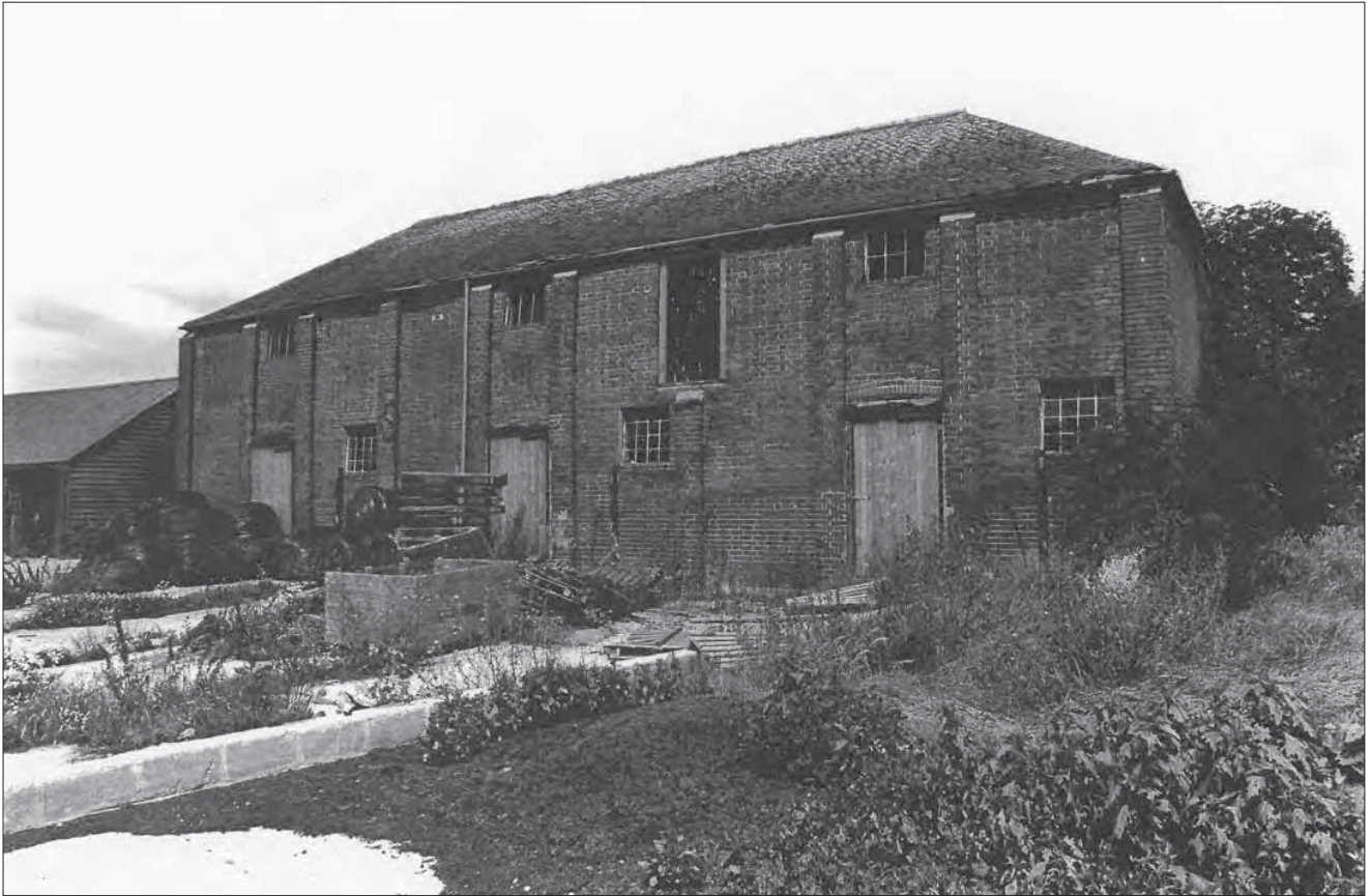
Appendix 4.8: Exterior view of the brick barn to the north of the farmyard viewed from the south east, taken in 2000 (image slightly cropped top/bottom). © English Heritage NMR Ref.: AA030276.
