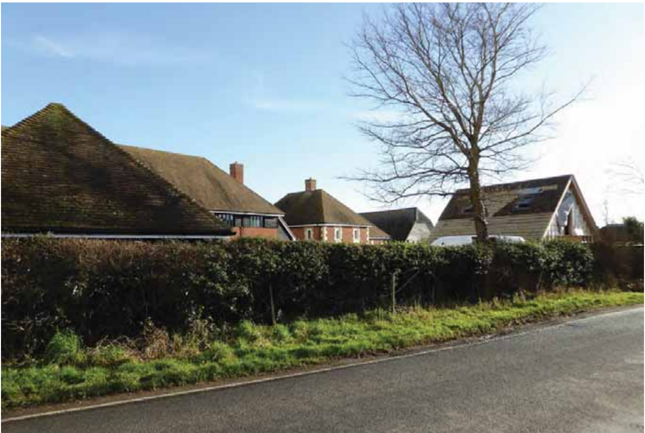
Appendix 8.2: The roof of the southern barn, framed between modern houses, from the north-west on Posbrook Lane, near Barn Close.
