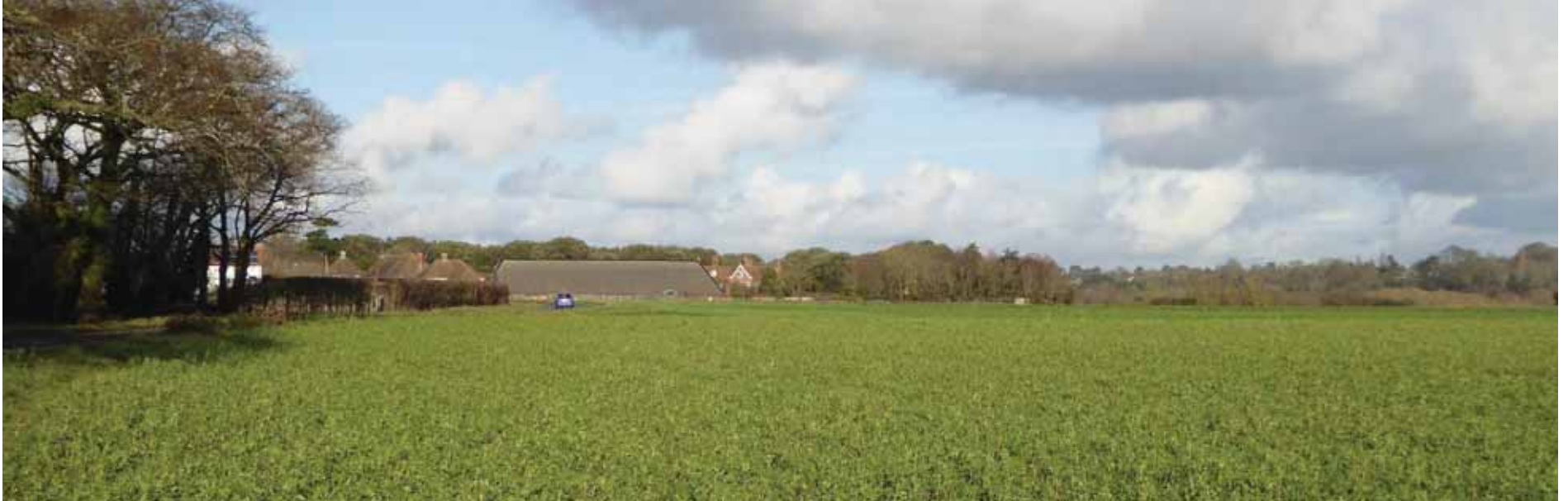
Appendix 8.9: The southern barn, seen in a long view from the south-west, on Posbrook Lane, near the northern end of the tree belt on the west side.
