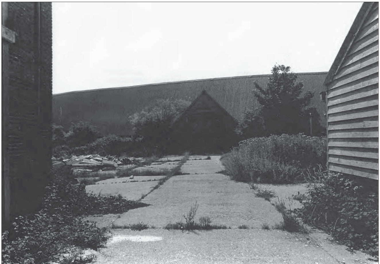
Appendix 4.9: Exterior view of the southern barn from the north, taken in 2000 (image slightly cropped top/bottom). © English Heritage NMR Ref.: AA030277.
