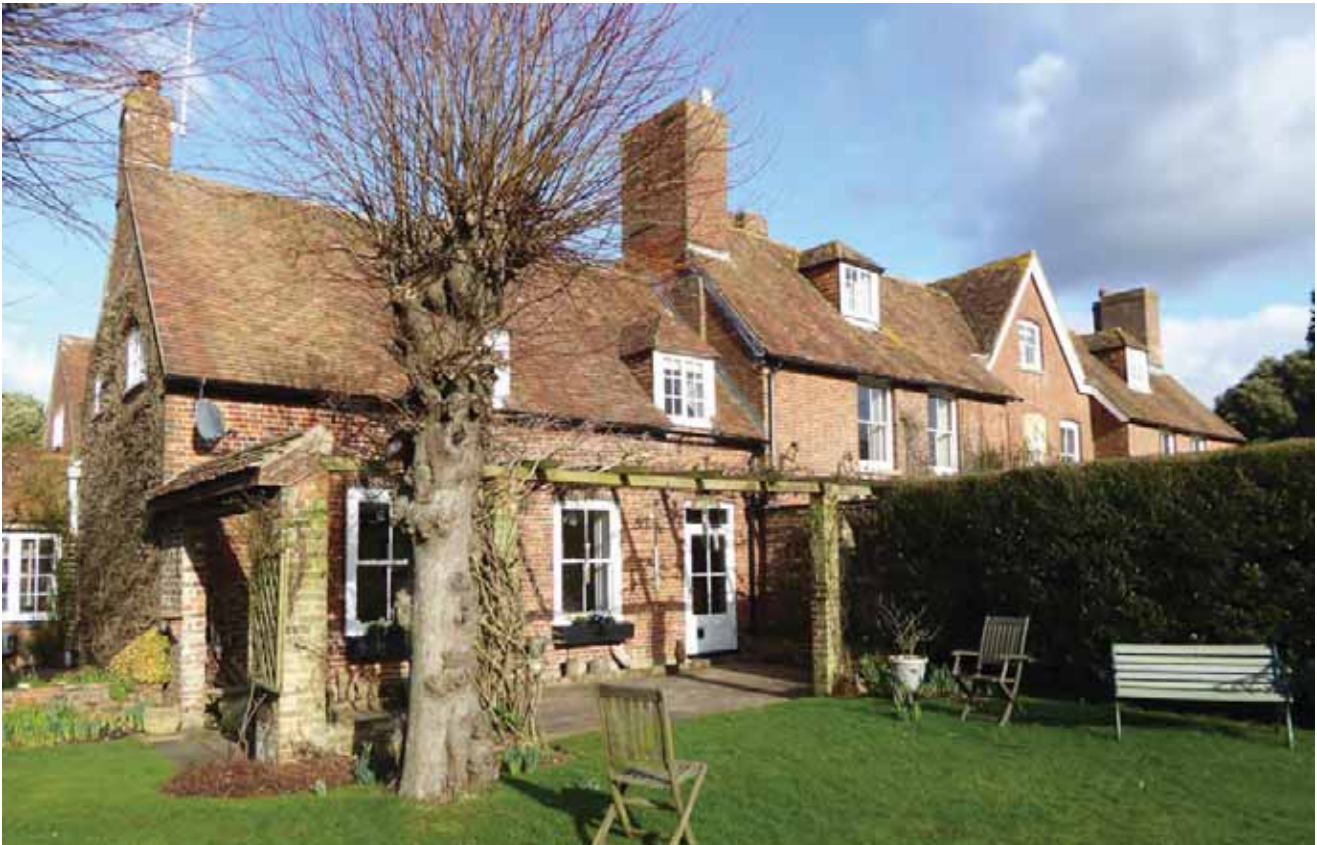
Appendix 6.6: Oblique view of the south façade of Great Posbrook from the south-west (the garden of Old Barn Cottage).
