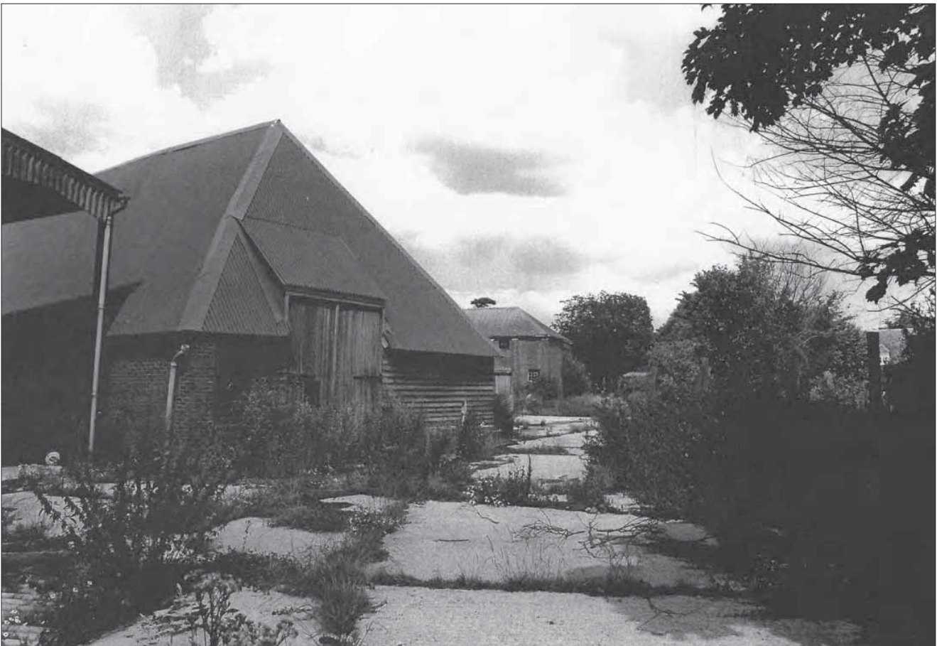
Appendix 4.5: Exterior view of the southern barn from the south-east, taken in 2000 (image slightly cropped top/bottom). © English Heritage NMR Ref.: AA030273.
